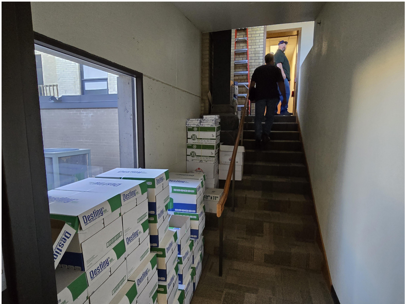
ADA Compliance (Elevator, lift, or ramp required - lack of proper storage)
