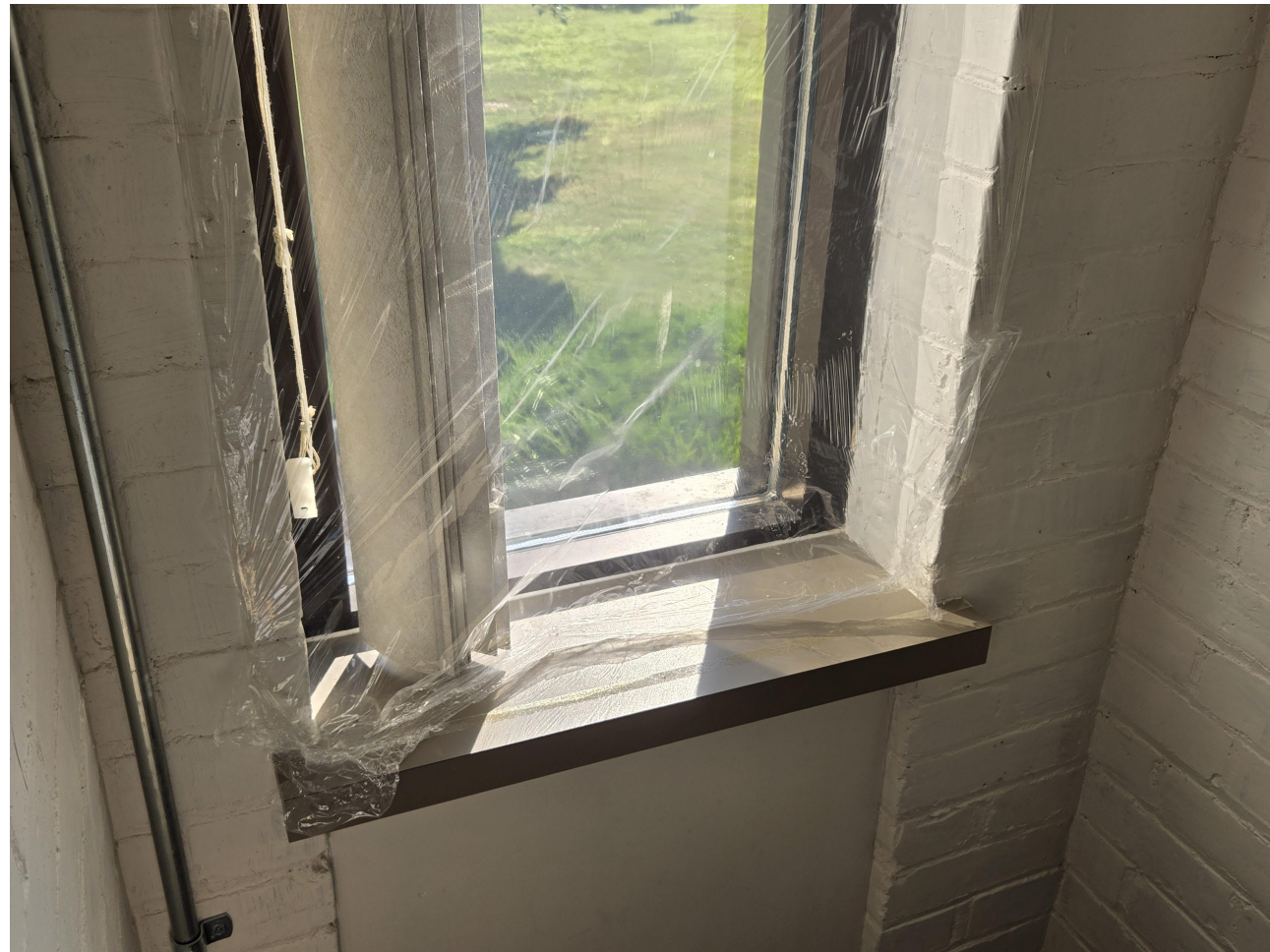
Inefficient windows (Courthouse windows 25 years old)
